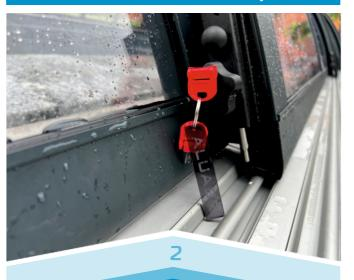
Our pool enclosures are equipped with a system of locks and special latches for the safety of children under 5 years old. It's made in accordance with European standards. Doors have special locks with a key. To open laches on segments you have to make two different movements at same time.
